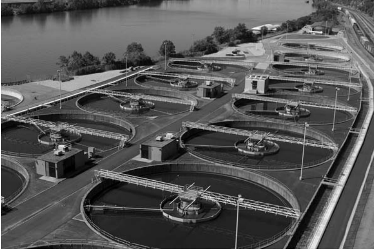
FIGURE 5.4 A typical water treatment facility. (Courtesy of Shutterstock.com.)
